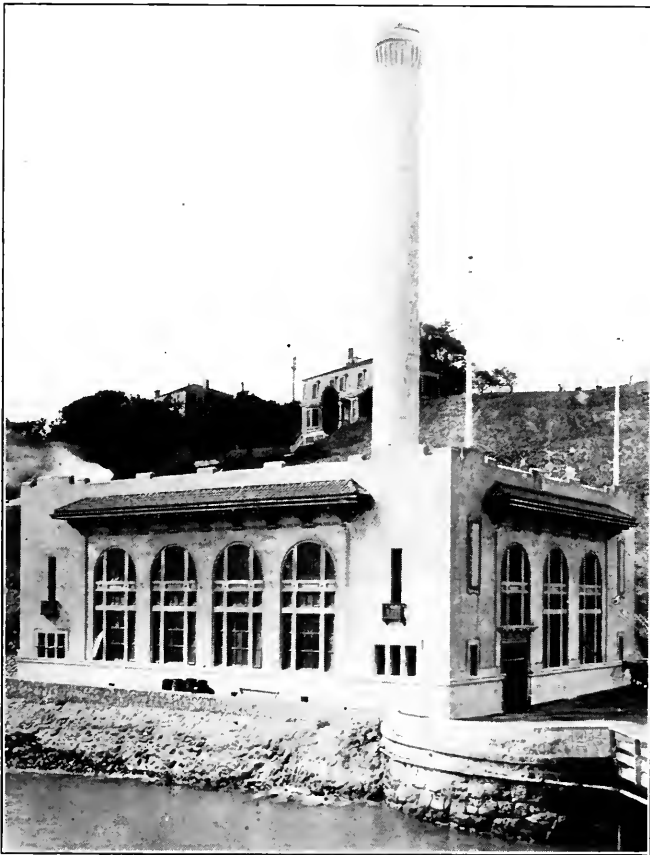
FORT MASON PUMPING PLANT
